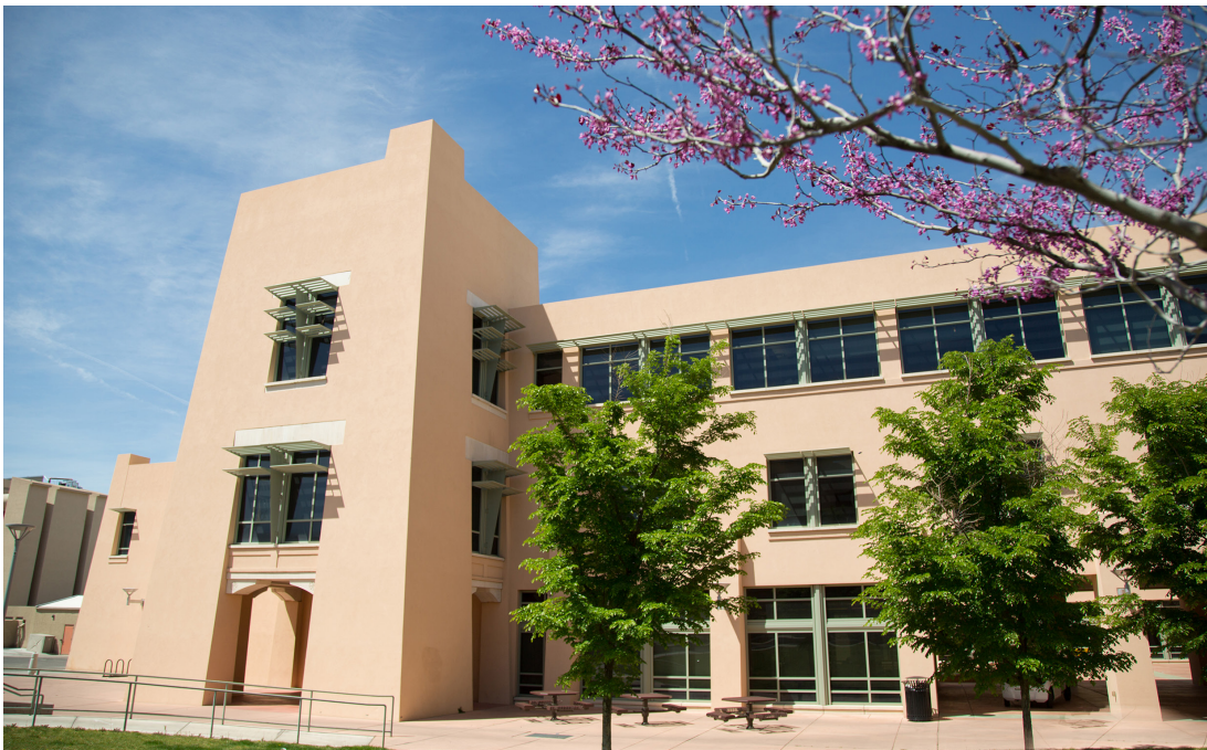
Centennial Engineering Center
